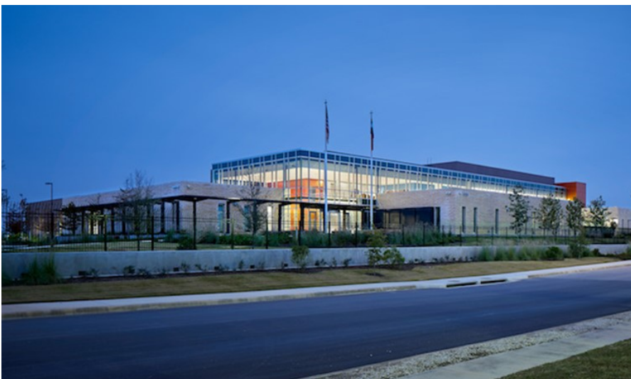
The Operations Center, which sits on a 9.4-acre lot, this summer will start serving as a backup for the city of San Antonio. Image: Courtesy of Page
